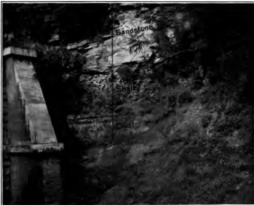
B. UPPER FREEPORT COAL WITH OVERLYING SHALES AND BASE OF MAHONING SANDSTONE AT SOUTH PORTAL OF BALTIMORE AND OHIO RAILROAD TUNNEL, STONY CREEK.
